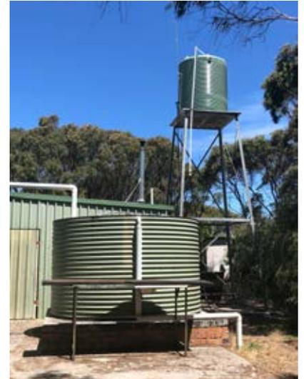
At the end of each stay the header tank must be refilled. This can be achieved when power is available – see Power section. A pump, located at the main tank, is used to fill the header tank. The main tap at the concrete tank must be open before the switch for the pump, located on the north wall of the shed (see picture above) is turned on.
